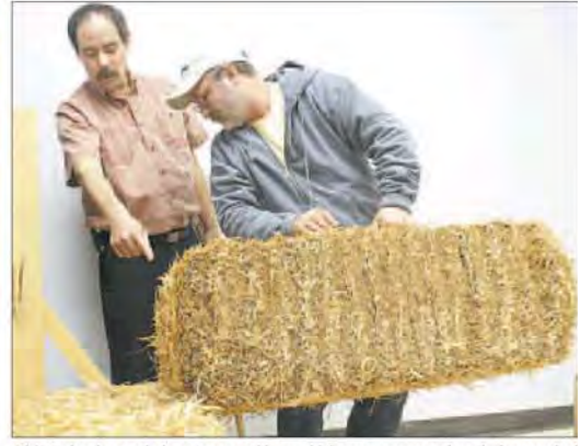
Kirk Taylor drops a bale onto a wood base which covers concrete foundation; vertical pegs with sharpened points skewer the bale into place.
