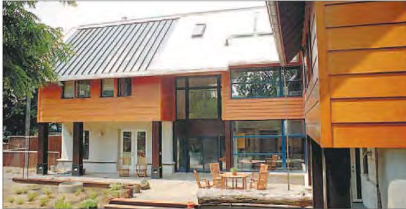
A straw-bale multi-family house provides excellent indoor air quality and a non-toxic environment.
